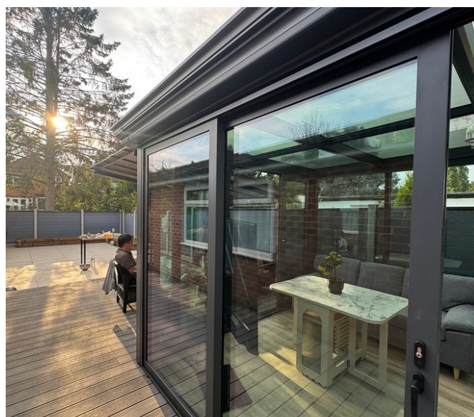
Façade and frame detail
