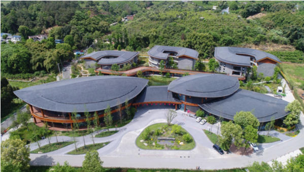
Location: Urban Education Practice Base in Chengdu Park Installed capacity: 130kW Application: Solar roof slate
