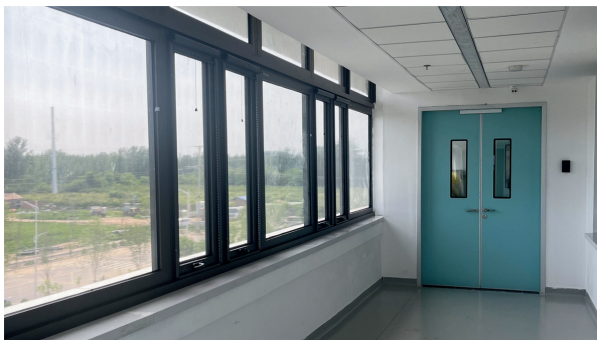
Location: BIPV Project for People's Hospital in Xiong'an New Area Installed capacity: 563kW Application: Casement window
