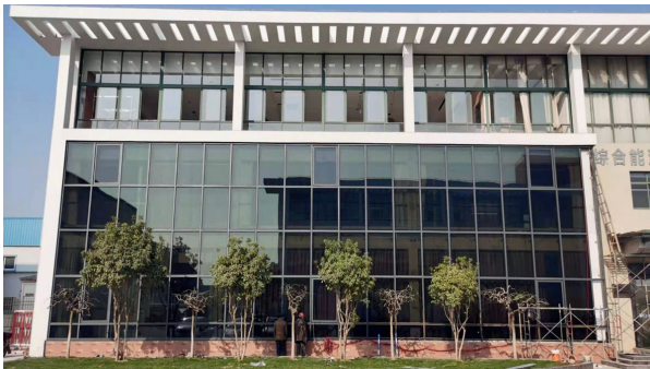
Location: Yancheng Comprehensive Energy Service Center Installed capacity: 10.44kW Application: Glass curtain wall
