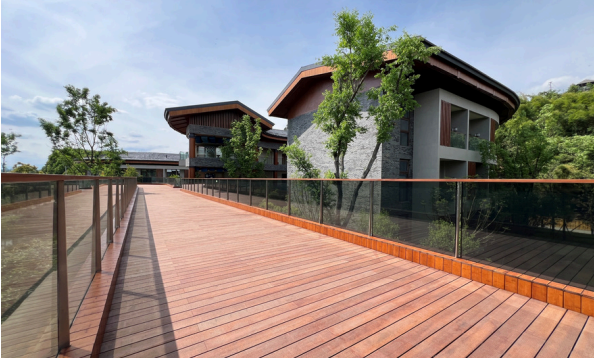
Location: Urban Education Practice Base in Chengdu Park Installed capacity: 130kW Application: Photovoltaic railing
