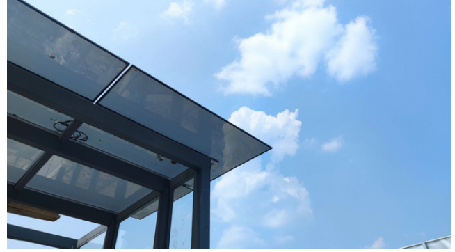
Location: Chengdu Jingyuan West Road Installed capacity: 32kW Application: Outdoor garage canopy
