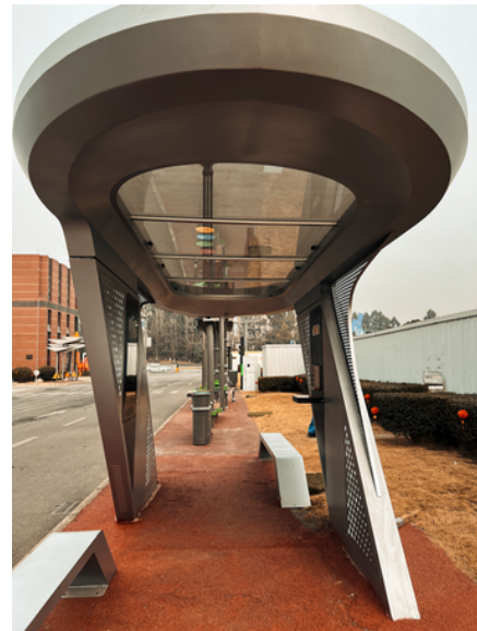
Location: Huati intelligent transportation energy storage station project Installed capacity: 0.75kW Application: Bus station Canopy
