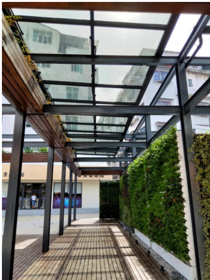
Location: Yijiashan Square Smart Community Installed capacity: 6.24kW Application: Corridor roof light
