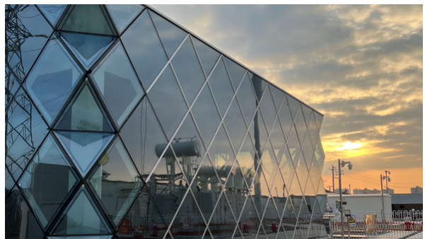
Location: State Grid Demonstration Project of New Power System Installed capacity: 99kW Application: Glass curtain wall
