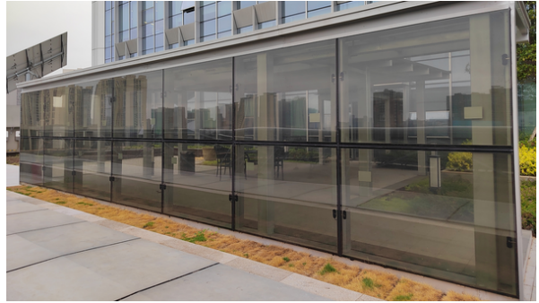
Location: Hunan Construction Engineering Sunshine Corridor Installed capacity: 2.38kW Application: Fixed Window
