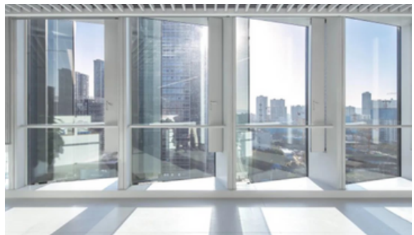
Location: Wuliangye High-tech Zone Headquarters Project Installed capacity: 346.5kW Application: Floor-to-ceiling glass
