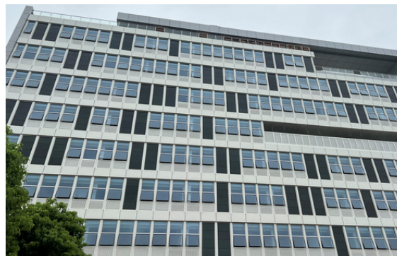
Location: Laboratory Building of Agricultural Biological Sciences, Academy of Agricultural Sciences Installed capacity: 78.82kW Application: Tilt & Down Window
